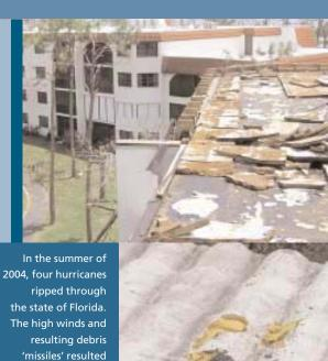
Roof decks encountering high winds can be damaged as a result of high-pressure differentials. When a door or window fails, this pressurization's effect on the roof increases, with dire consequences—the deck (and the roofing membrane) can quite literally blow up.
